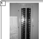
Before you begin installing the fan, Switch power off at Service panel and lock service disconnecting means to prevent power from being switched on accidentally. When the service disconnecting means cannot be locked, securely fasten a prominent warning device, such as a tag, to the service panel.
